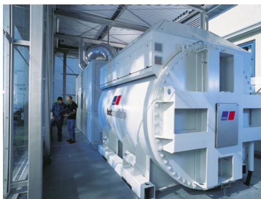
The first bi-fuel fuel cell. It is run with natural gas, methanol, or both.
